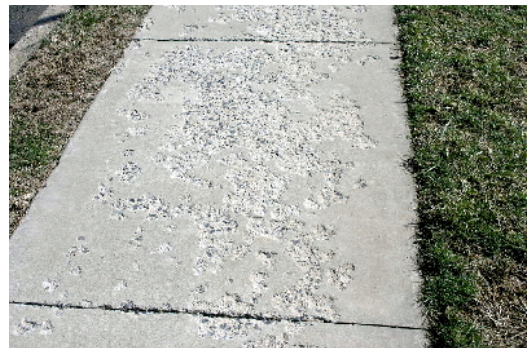
Spalling associate with salt damage.
