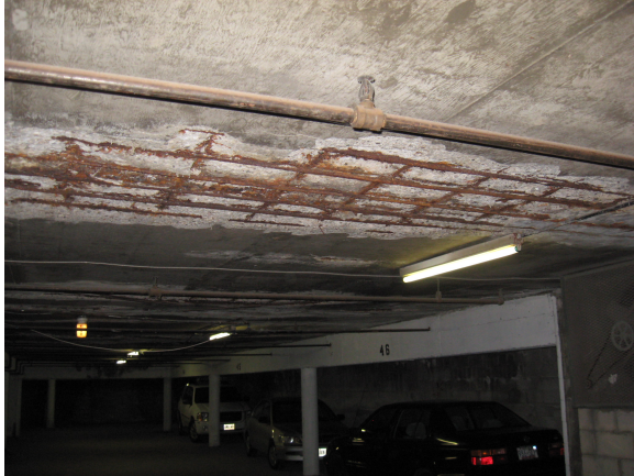
Reinforcement exposed due to carbonation. Shallow placement of the rebar accelerated the corrosion.
