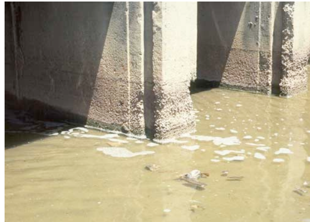
Sulfate attack on bridge supports over a run-off canal.
