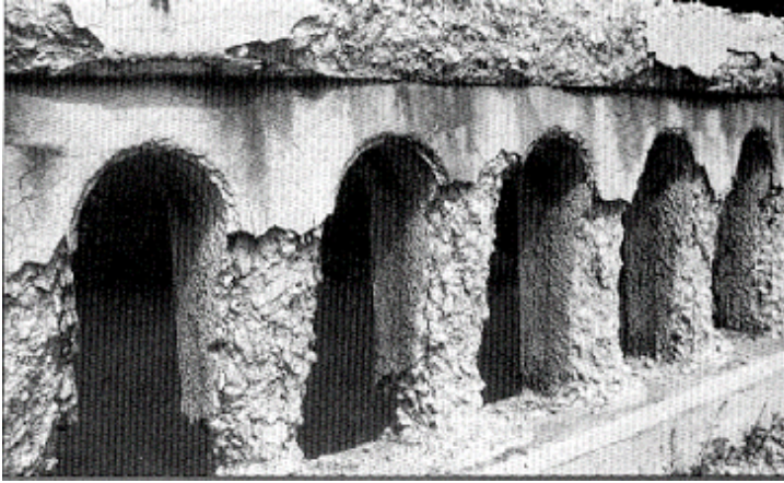
Freeze/Thaw damage to a bridge support. Pressure created from freezing water has “exploded” the surface of the concrete.
