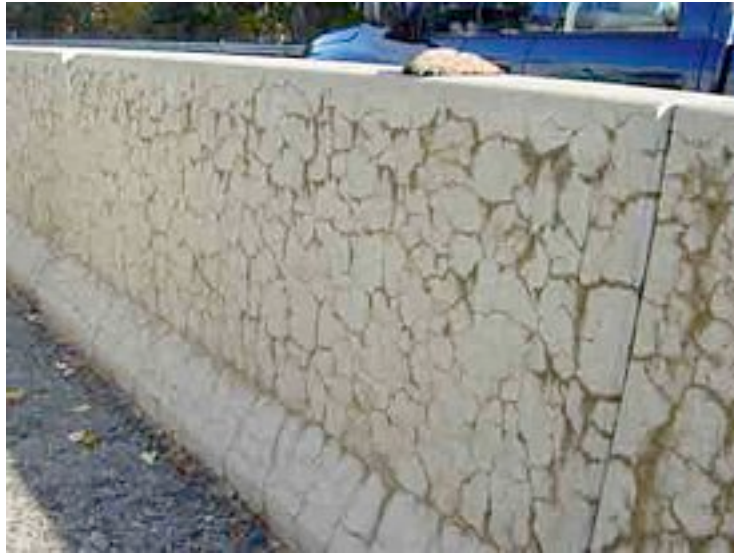
Alkali Silica Reaction (ASR) on a highway divider.
