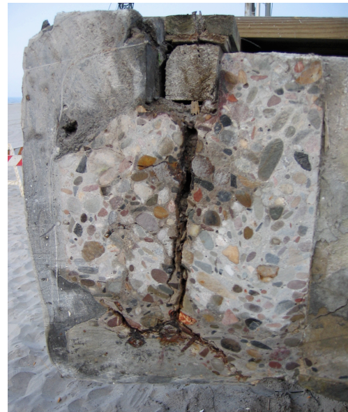
Structural failure of concrete due to corrosion of the reinforcement.
